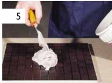
5 The packages are dosed to make no errors. The mixture is workable for about 45 minutes at +23°C.
