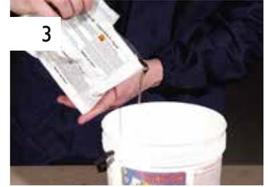
3 Pour all the catalyst (component B) in the component A.
