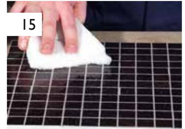
15 Seal the tesseras and remove the excess mixture from the tile.
