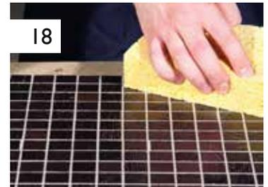
18 Remove the mixture from the tesseras, without emptying the groutings, and drying the excess water.
