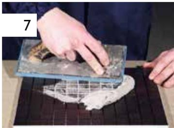
7 Stick the mixture in the tile groutings, with a rubberized flat trowel.
